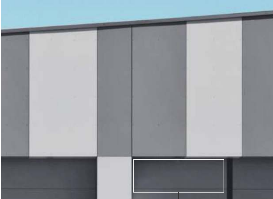
Dummy modules used to cover the shaded parts.
